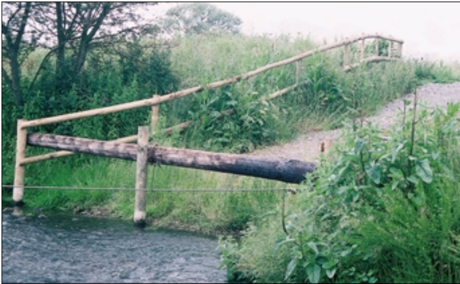
Stock watering point at ch. 100m
