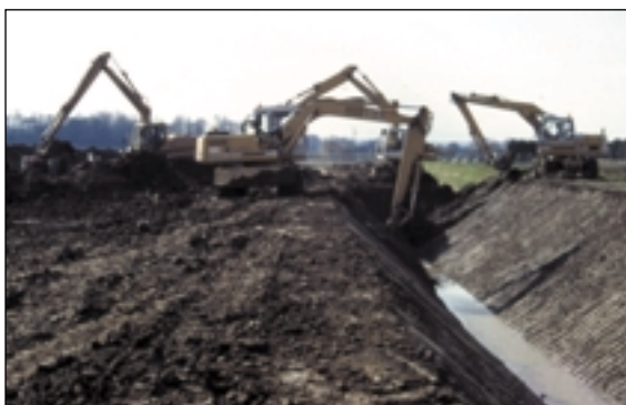
Relocating the IDB drain and set-back floodbank
