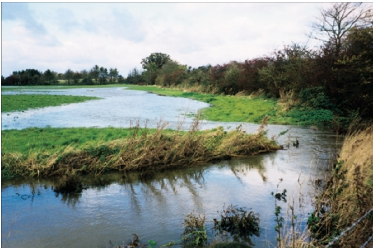
Spillway S4 . Floodwaters spilling into field gully.
