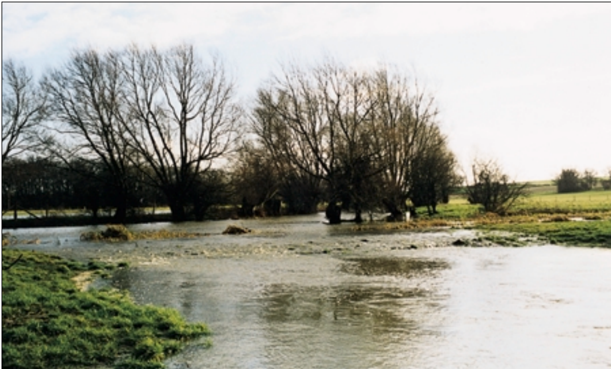
Spillway S2 in flood
