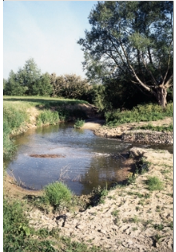
Gabion weir and pool
