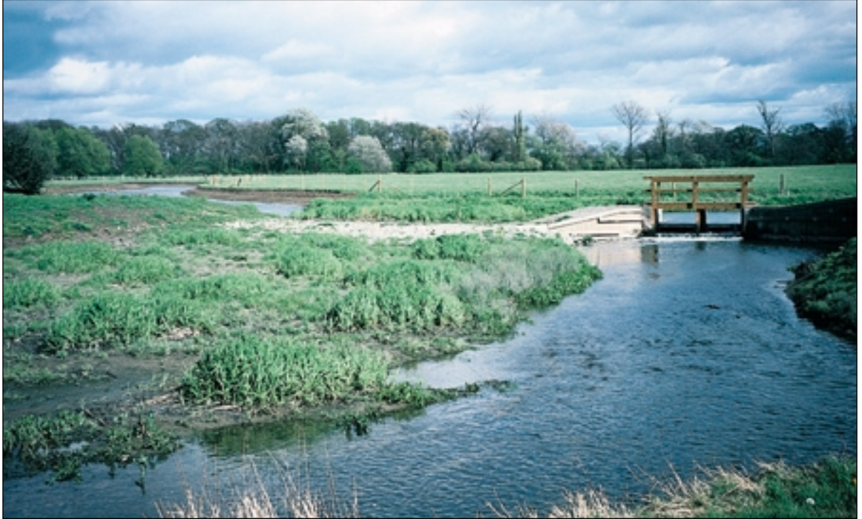
Spillway alongside bifurcation weir – April 1997
