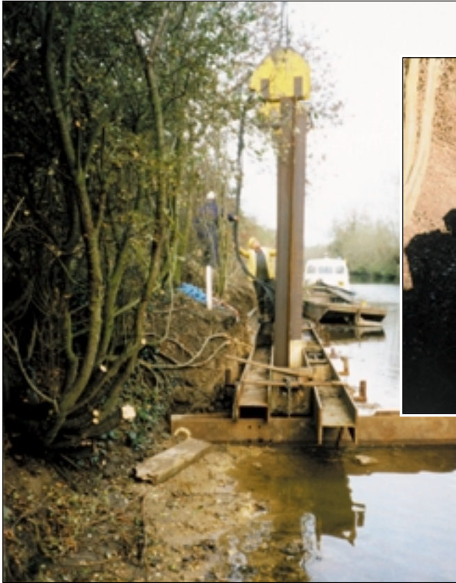
Initial sheet piling after bagwork removal, over existing trees
