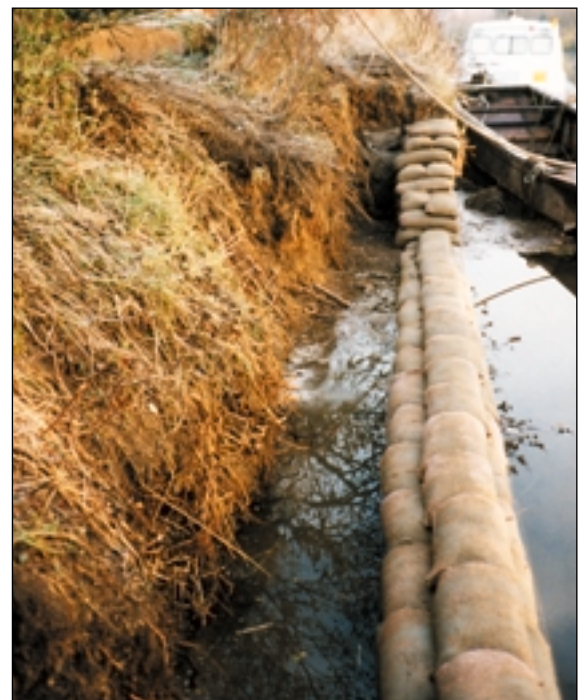
2 layer capping bagwork and tie-in to existing sheet piling
