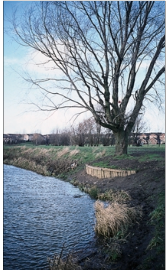
Protected roots after work completed – February 1997
