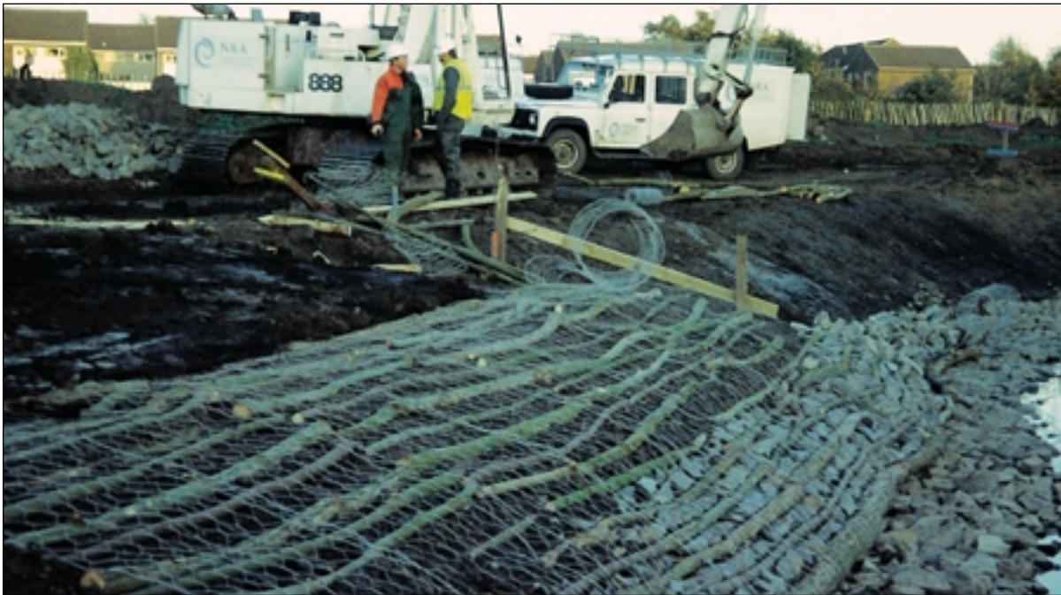
Mattress revetment under construction – October 1995
