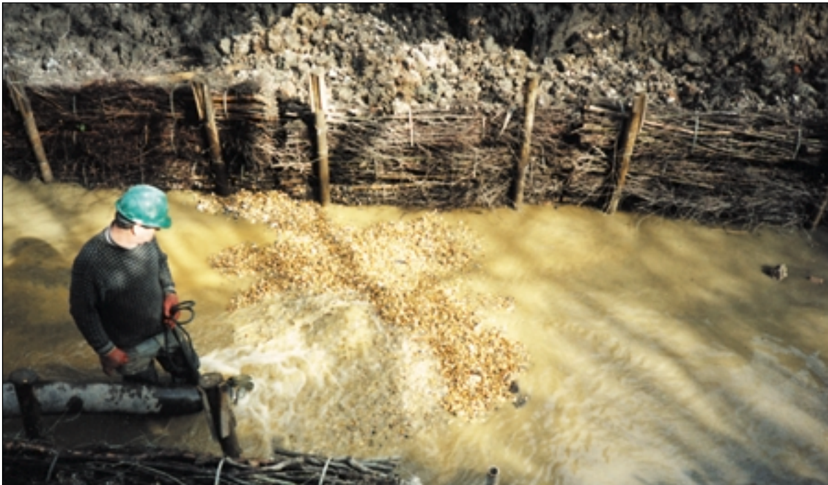
Gravel pumping in operation
