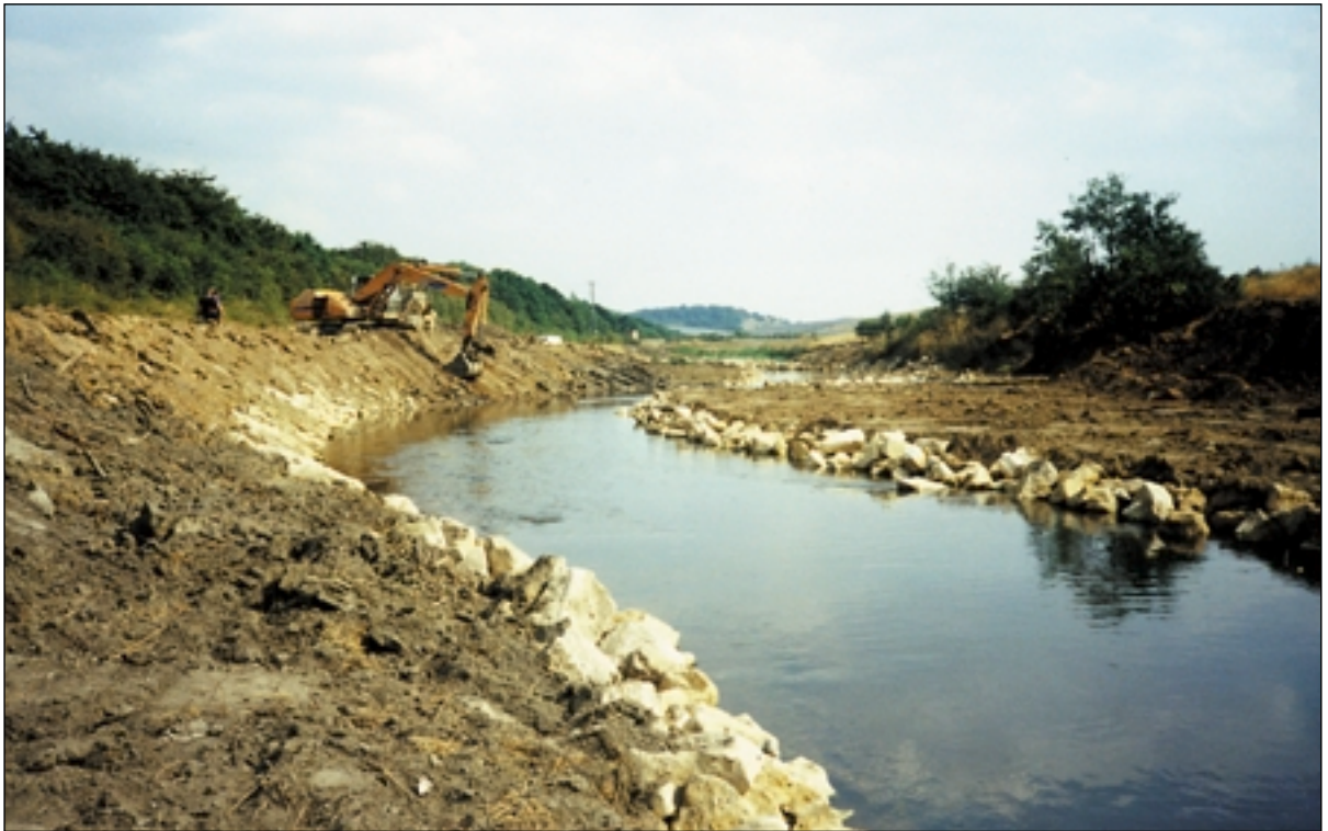
Placement of limestone boulders and berm back-filling
