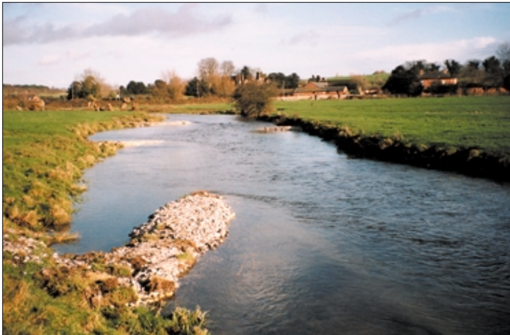
Completed chalk groynes
