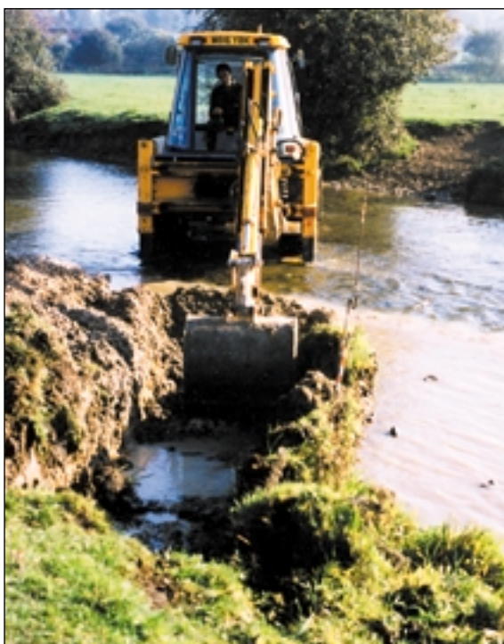
Digging the groyne trench
