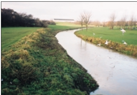
View downstream before deflectors constructed
