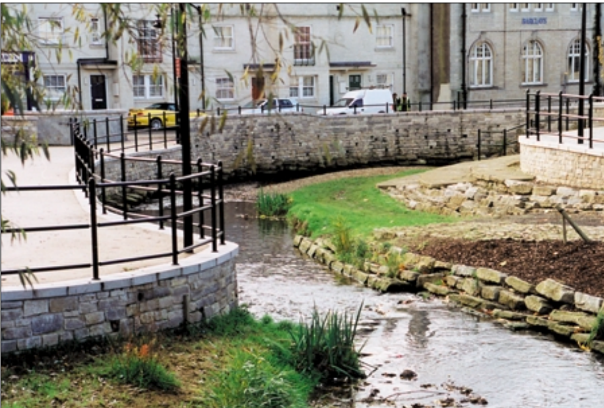
View of Section A in November 2001
