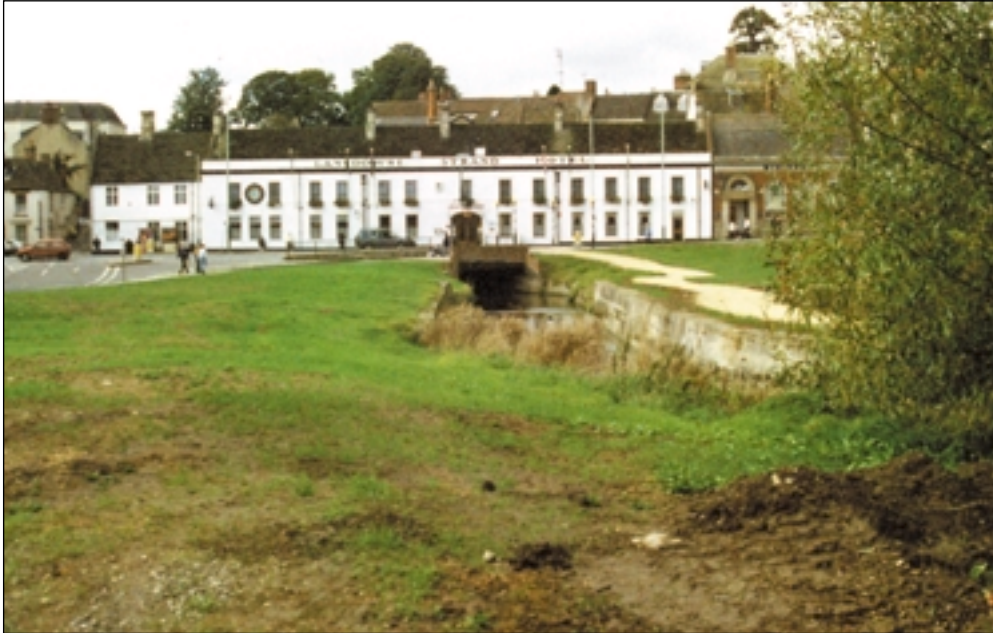
Before: View downstream towards culvert
