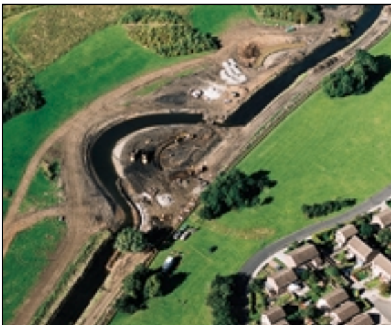
Meander excavation – Autumn 1995
