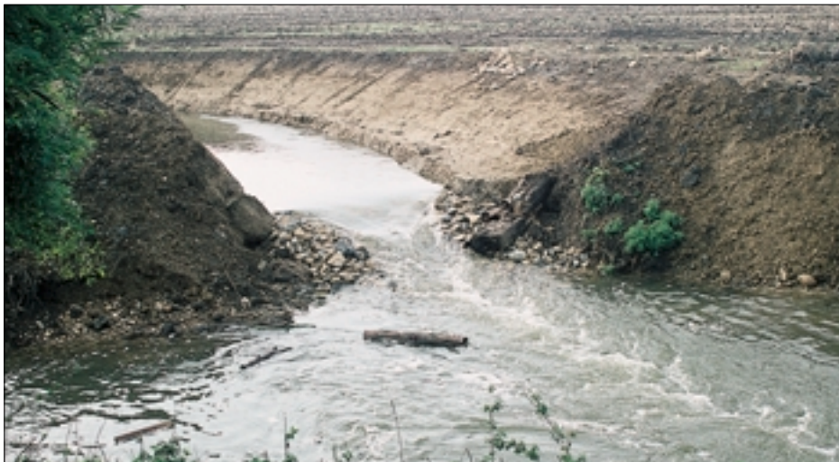
New channel flowing into existing channel during construction – September 1995
