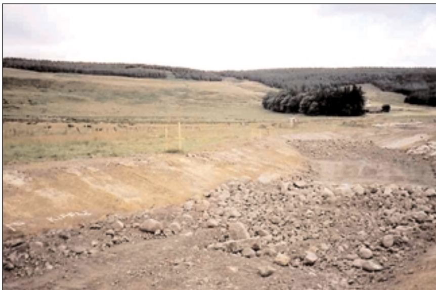
Shaping the new channel within the clay lining
