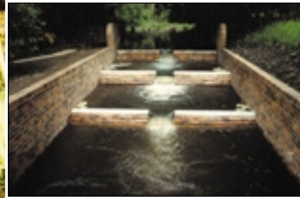
Mill weir and replacement fish-pass
