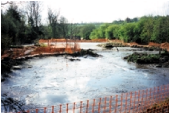
Dewatering – April 1995. View from inlet channel
